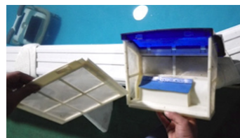
5. Pull out the filter panel vertically
