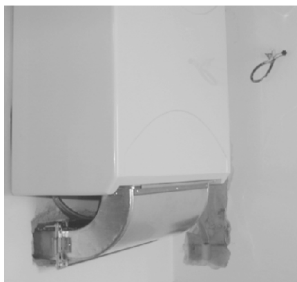
View from the adjacent room
