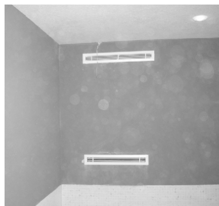
View from the swimming pool hall
