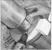
Strap the duct clamps on each side of the fan with the screws.
