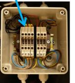
Picture: Four pin terminal connection of water unit (1-4 sensor connection with condensing unit) and three pin terminal connection of the control display (A,B,C).
